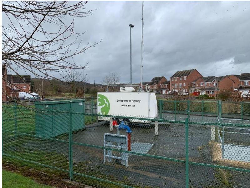
Above: The Mobile Monitoring Facility (MMF) in the grounds of the Severn Trent Pumping Station off Galingale View.
